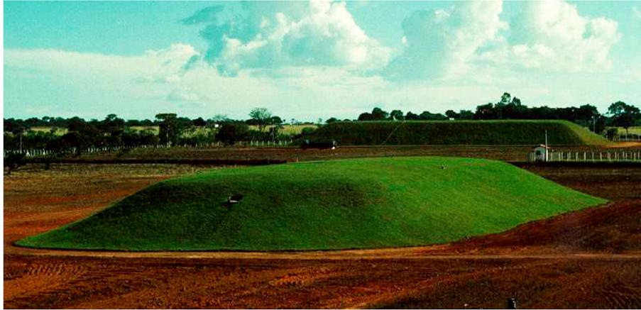
**Fig. 1.** View of the Goiânia near-surface repositories. The repository in the front contains relatively low-activity  $^{137}\text{Cs}$  waste (specific activities less than 87 Bq/g), and the repository in the back higher-activity waste (specific activities above 87 Bq/g).
